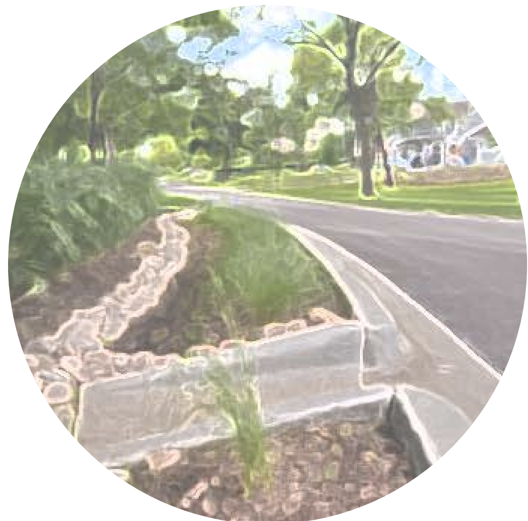
Stormwater Planters and Parkway Bioswales
